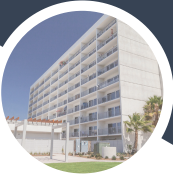
KIMBALL/MORGAN TOWERS Community HousingWorks SENIOR-LIVING
